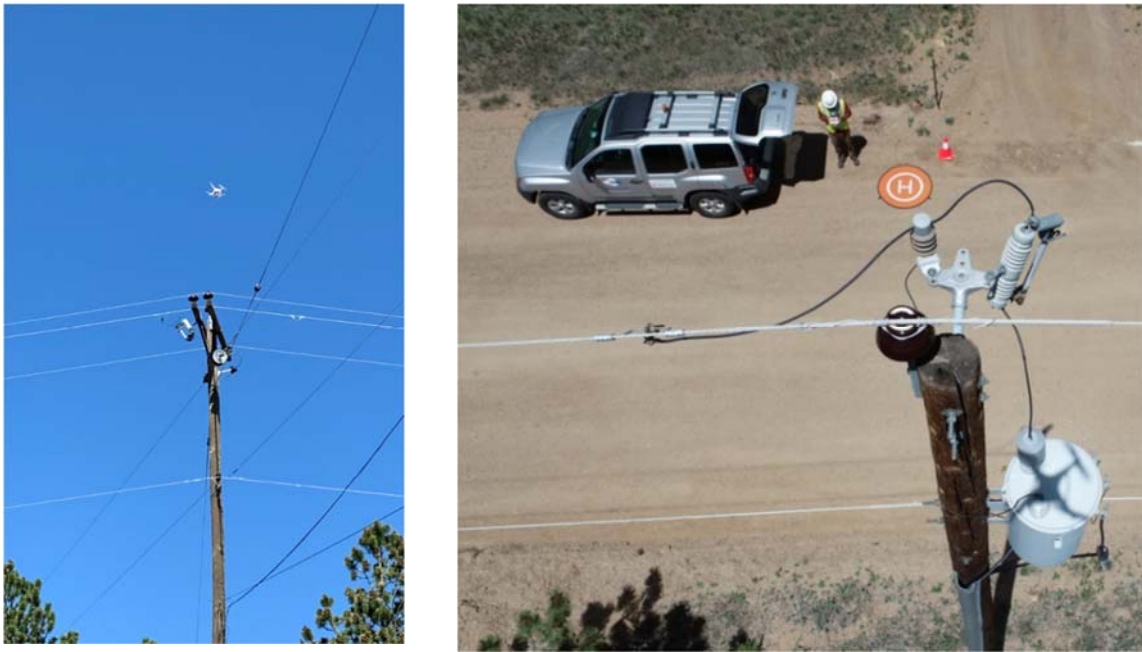
Figure 6-5: UAS Pilot Collecting AGL Inspection Imagery
