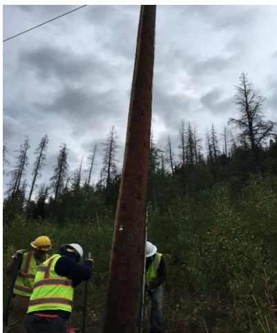
Figure 6-1.: Inspection crew excavating a pole in mountainous area
