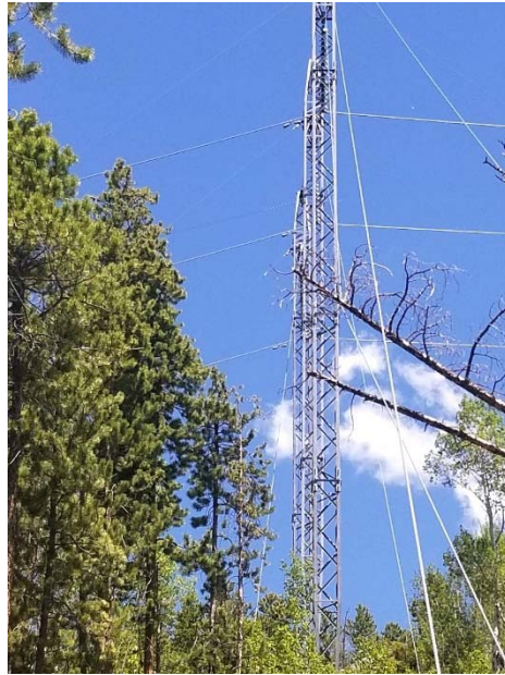
Figure 6-13: Example of Hazard Tree
